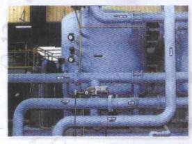
port valves are normally used. Automatically backwashed filters use butterfly, diaphragm and multi-port valves with electric, hydraulic, or pneumatic actuators.
